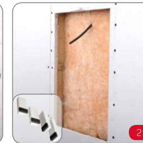
2 Position installation lugs under top and bottom corners of surrounding plasterboard. Ensure cables are pulled to this position.
