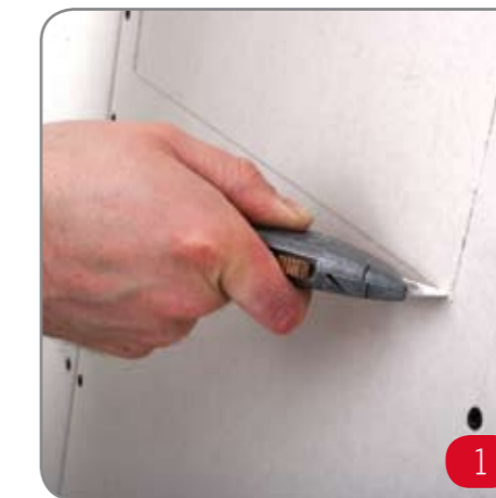
1 Create aperture using a sharp knife, making a series of shallow cuts. Add sound insulation into cavity.
